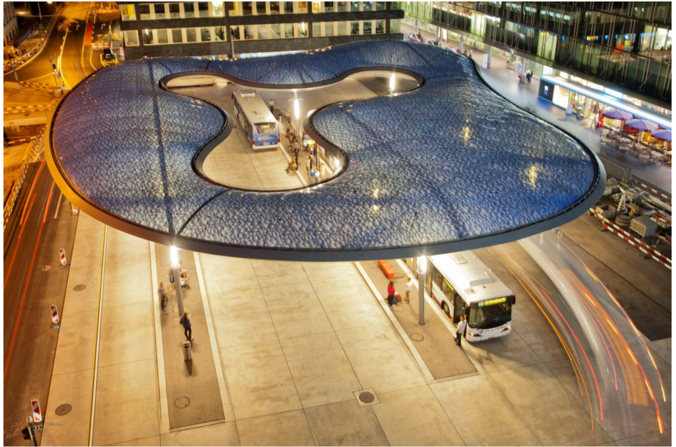
Canopy Bus Terminal Aarau / vehovar & jauslin / form TL / Arge Foliendach RUCH AG + Vector Foiltec © Niklaus Spoerri
