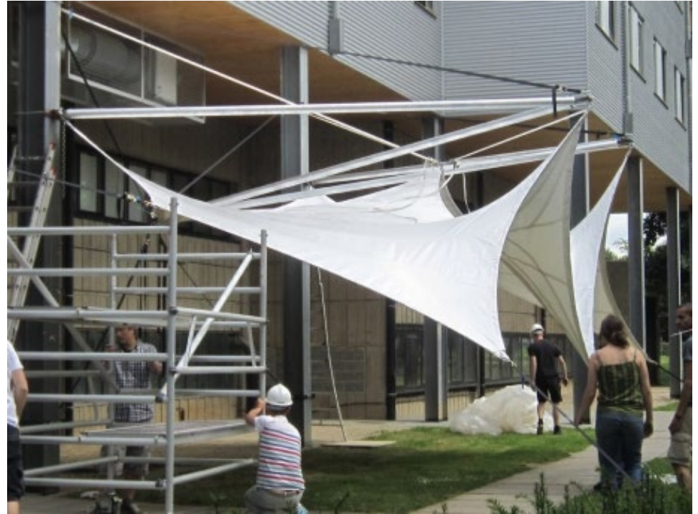
Students at VUB during erection of lightweight structure
